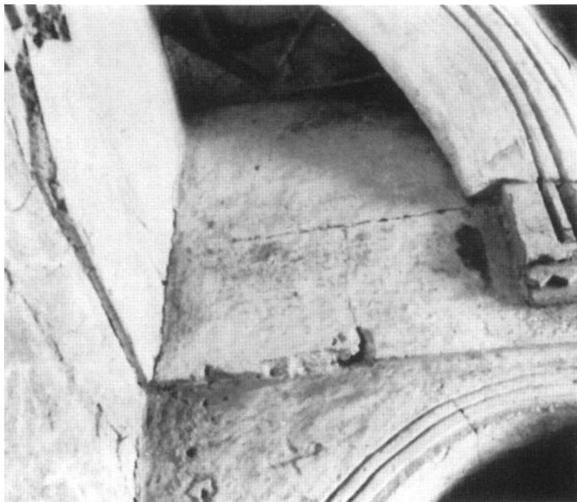
b. Squinch arch in upper room, with graffito inscription between the springing of the arch and the angle of the walls, dated 91/710.
