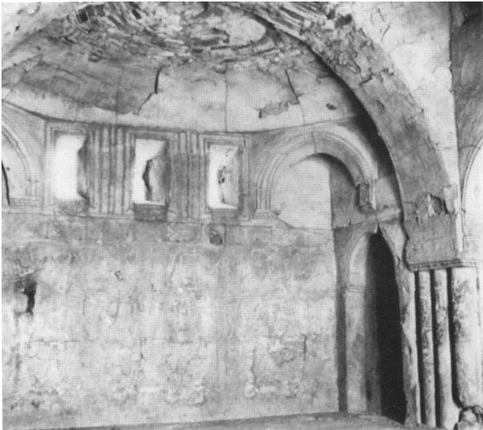
a. Upper floor room, with a semi-dome supported on squinch arches.
